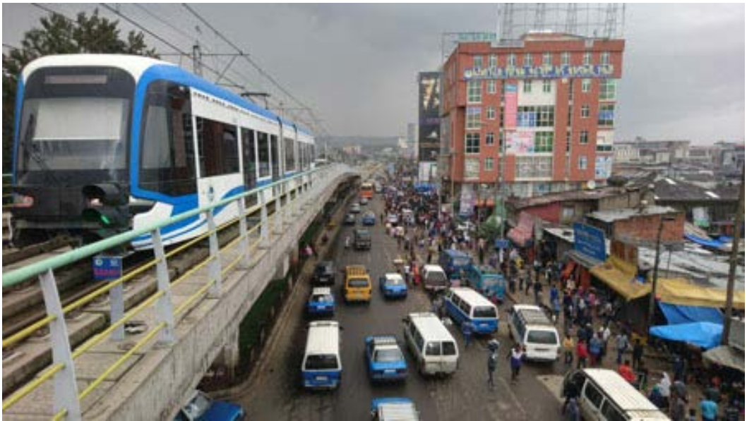
Figure 1. Addis Ababa’s Light Rail Transport System.
